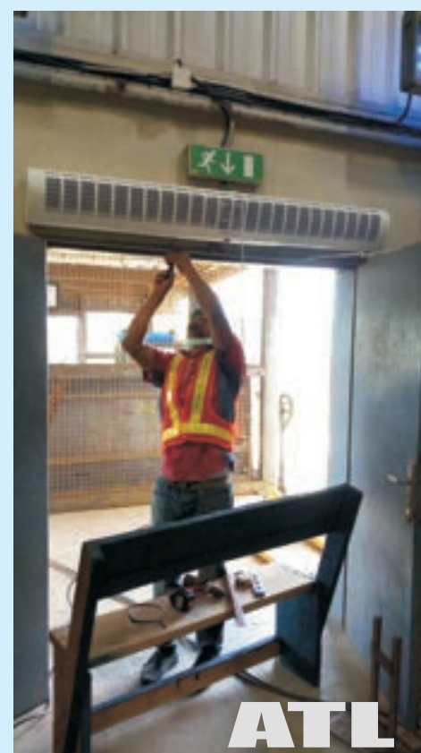
Importation and installation of air curtain Agbara, OPIC Estate.
