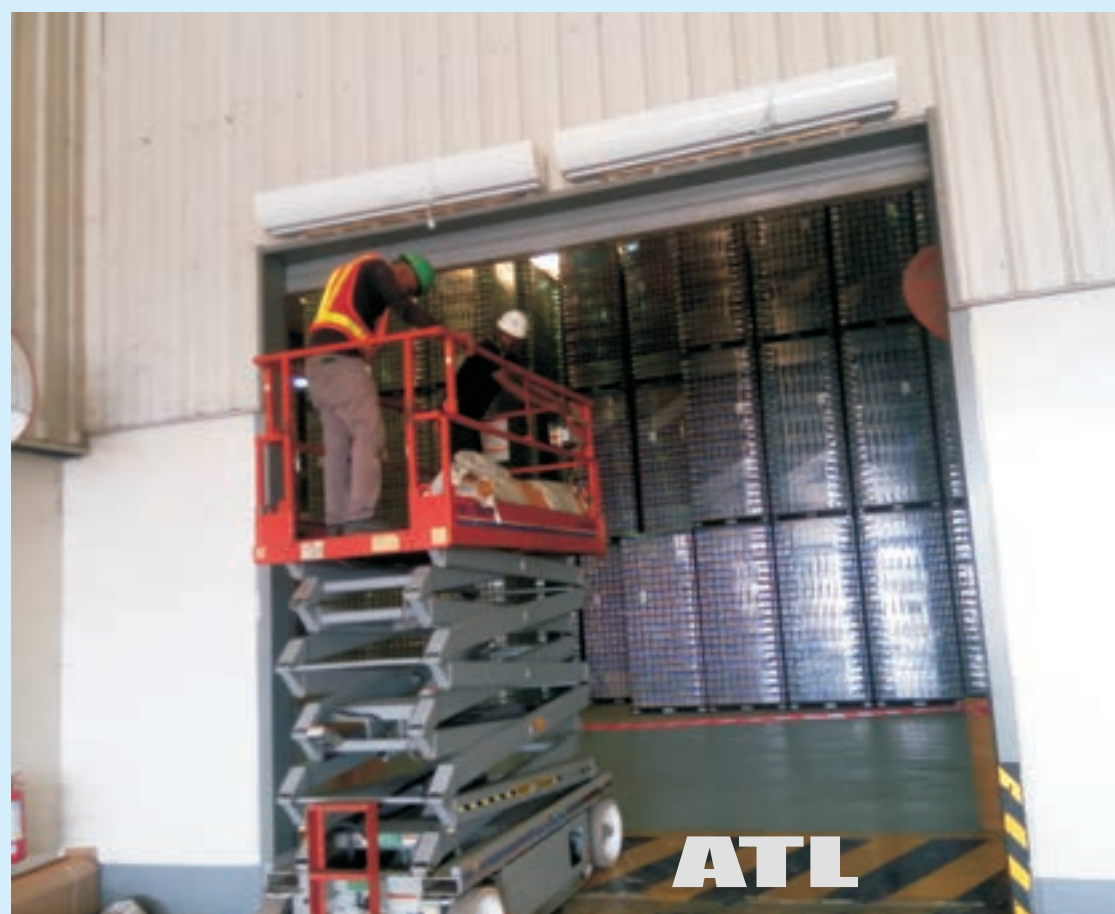
Importation and installation of air curtain Agbara, OPIC Estate.
